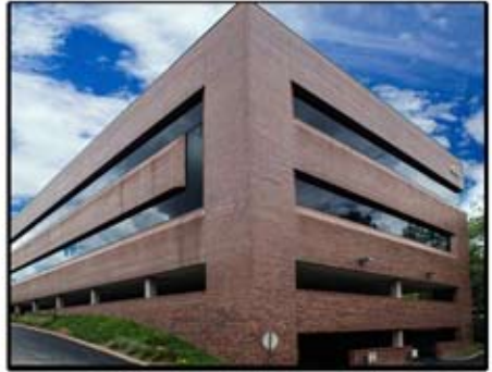
675 Old Ballas Medical Building Creve Coeur, MO 63141
